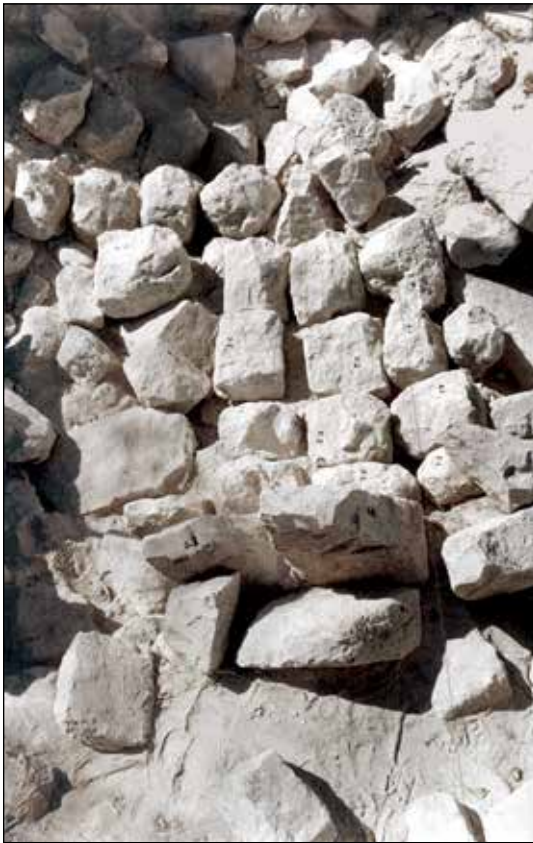
Figure 8. In situ facade stones in the excavation.
