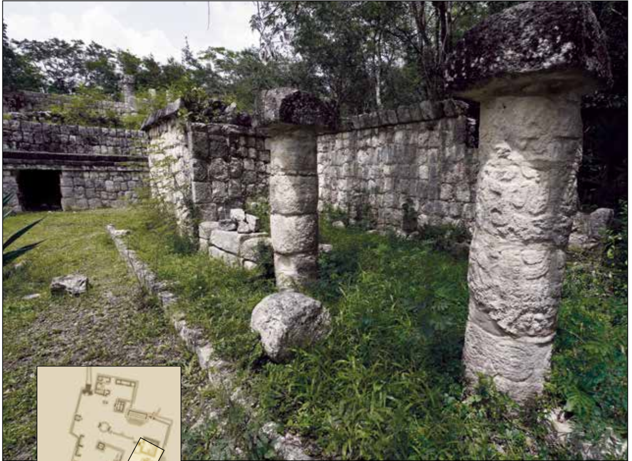
Figure A-14. The House of the Moon columns: view from the southwest.
