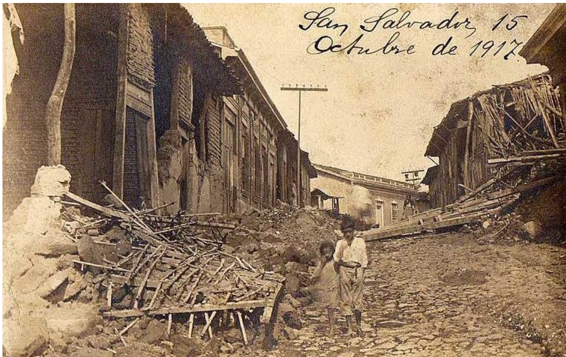
Figure 3.3. Postcard showing earthquake damage in San Salvador.
