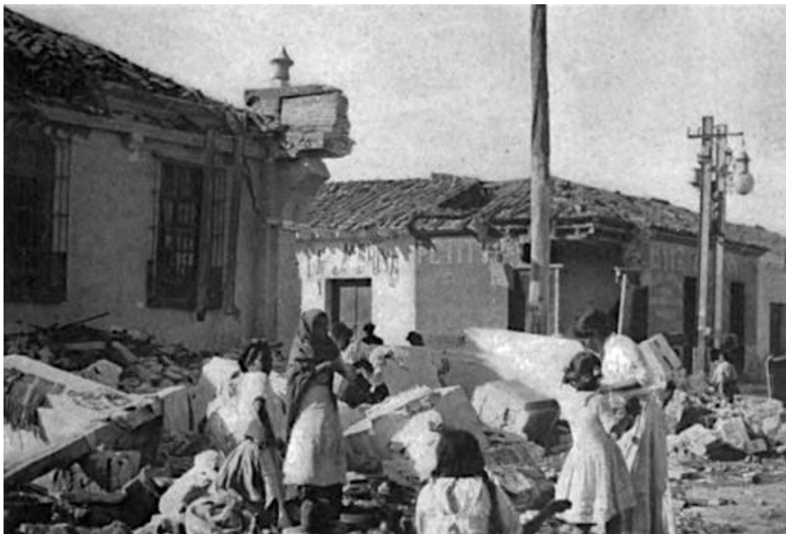
Figure 22.7. Morley's photograph of earthquake survivors gathered around a broken water main in front of the National Palace, in search of drinking water.
