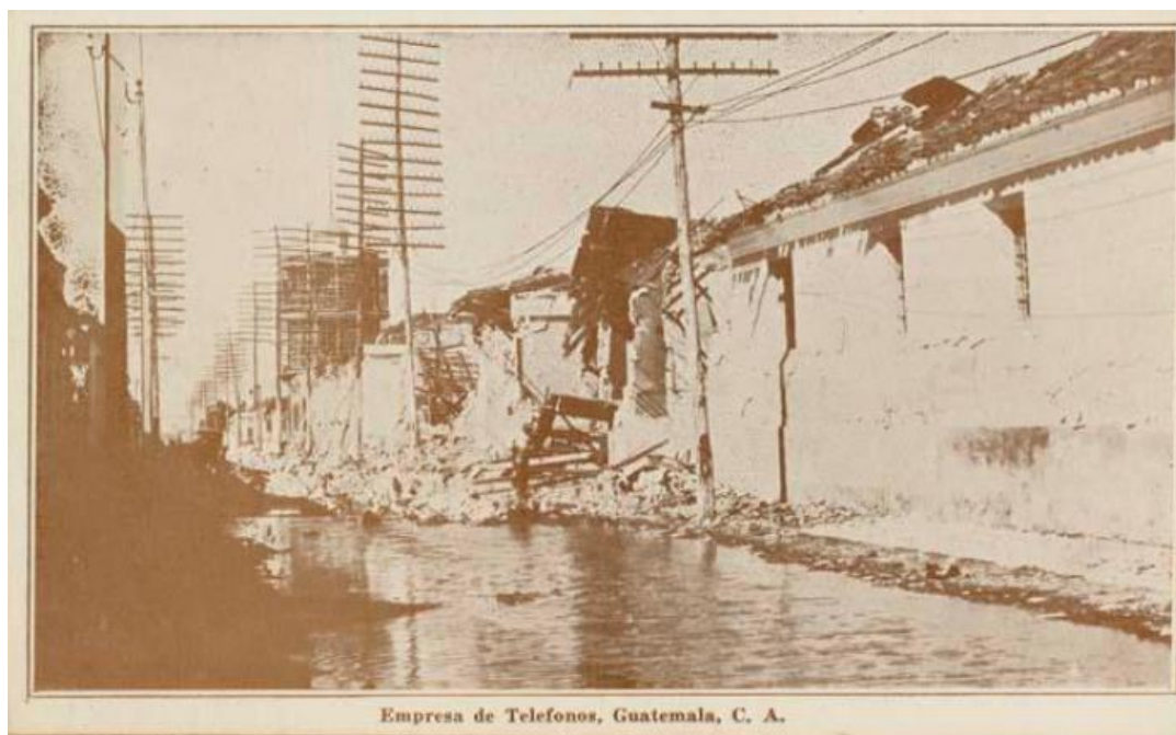
Figure 22.1. Postcard showing damage to the Guatemala City telephone office after the Christmas earthquake.
