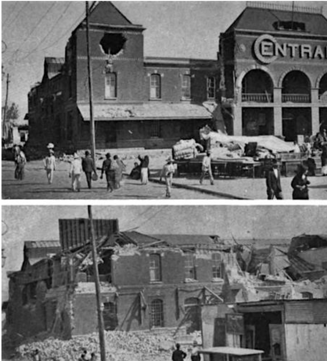
Figure 22.2. Two views of the train station, both taken by Morley. Top, the damage suffered by the December 25th quake; bottom, additional damage from subsequent quakes. Morley's temporary quarters were in the rail yard immediately behind this structure.
