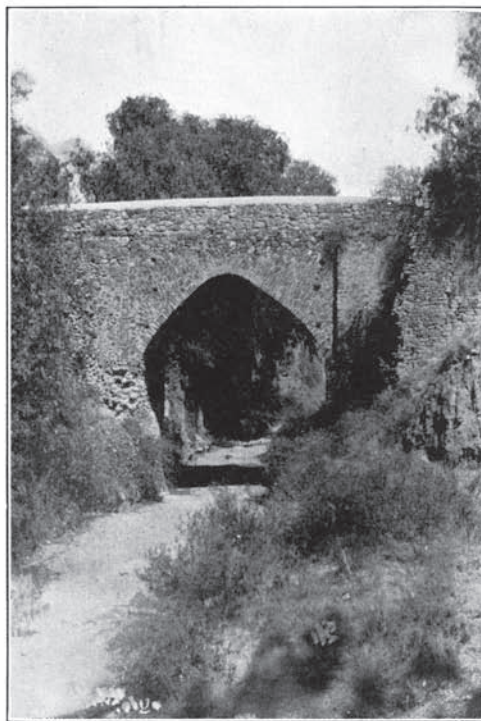
FIG. 7—Huexotla, D. F. Old Spanish Bridge.
