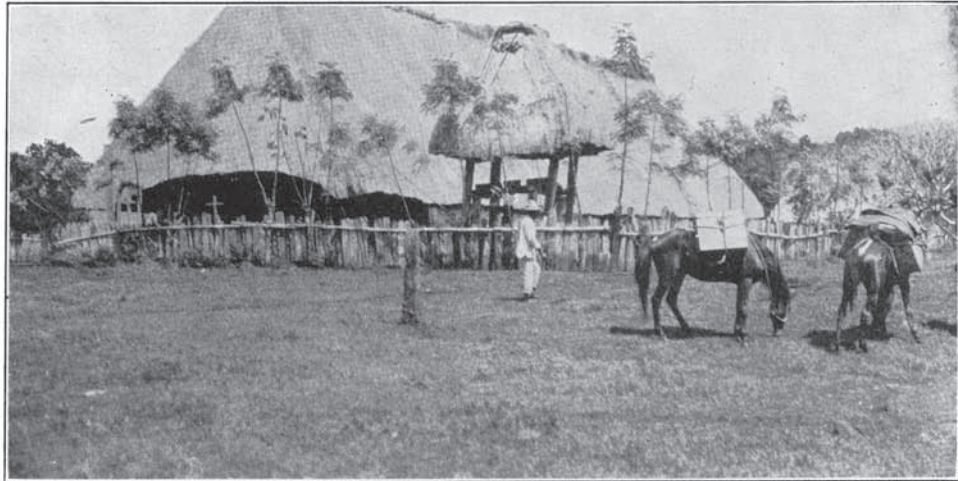
FIG. 31—Mecayápan, Ver. Church and Steeple.
