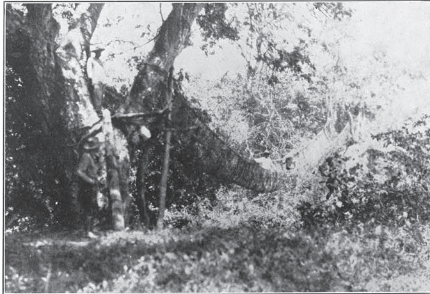
FIG. 32—Tatahuicapa, Ver. Hammock Bridge Made of Vines.
