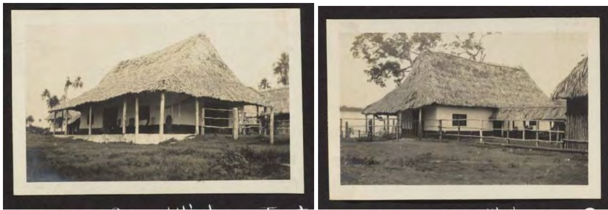
Figure 37.2. Shufeldt's well-made house that so impressed Morley.
