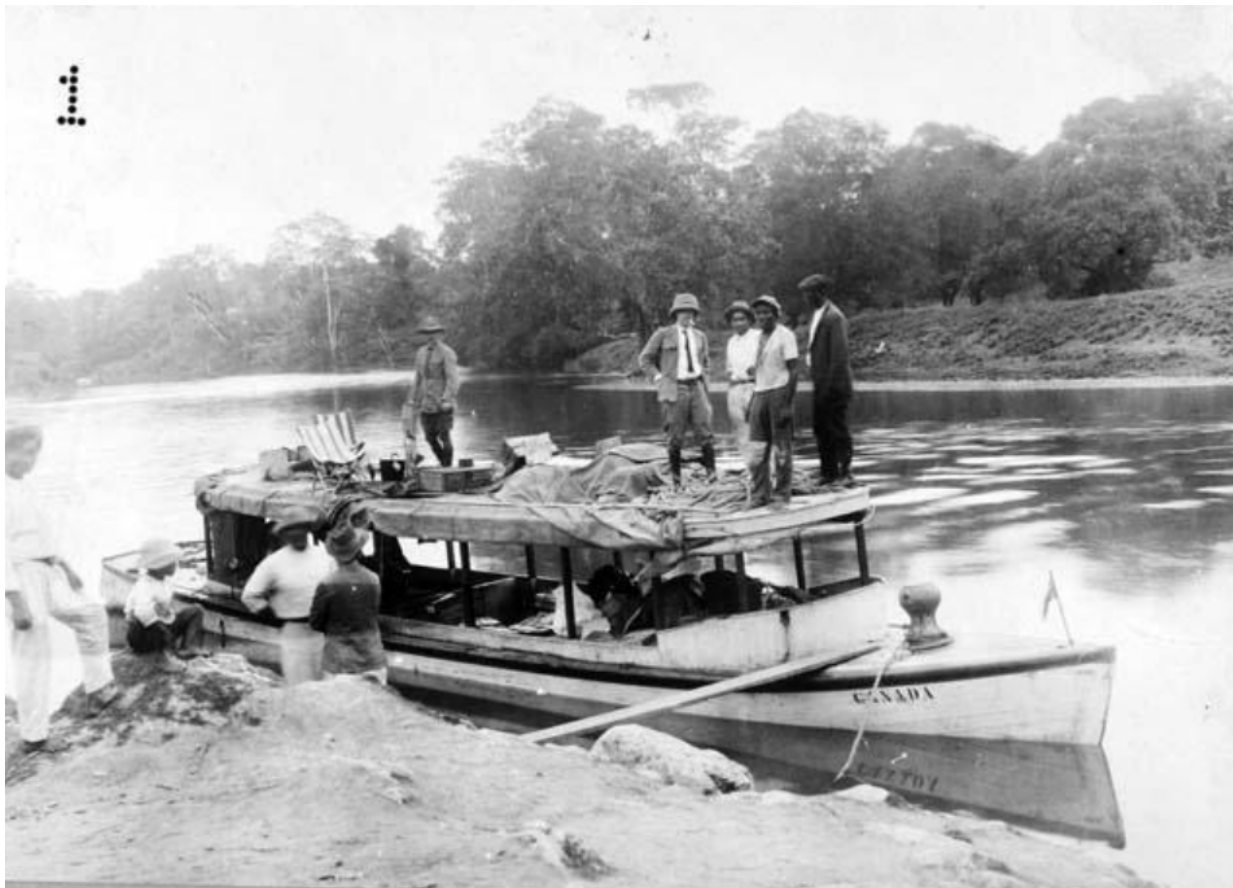
Figure 14.3. Morley (center with the white shirt and tie) and Ricketson (on the roof to the left) aboard the Canada .
