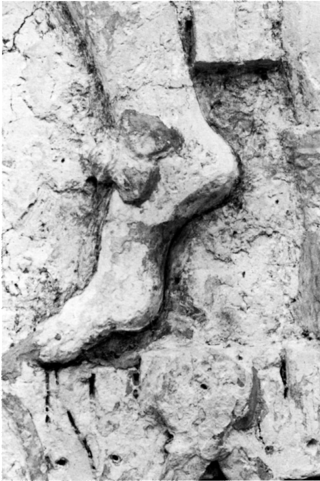
Fig. 7 Detail of clubfoot pier d, House D
