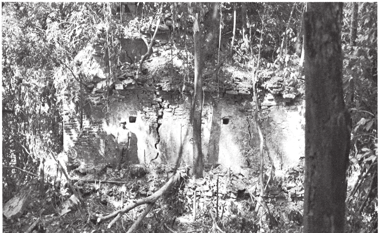
Fig. 2 South facade of the Olvidado showing rectangular openings
